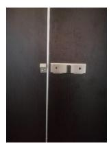
4.6.1.4.8 12 mm thk waterproof compact laminated board urinal partition including 0.5 mm stainless steel angle bracket with complete accessories. Approved type and quality.
